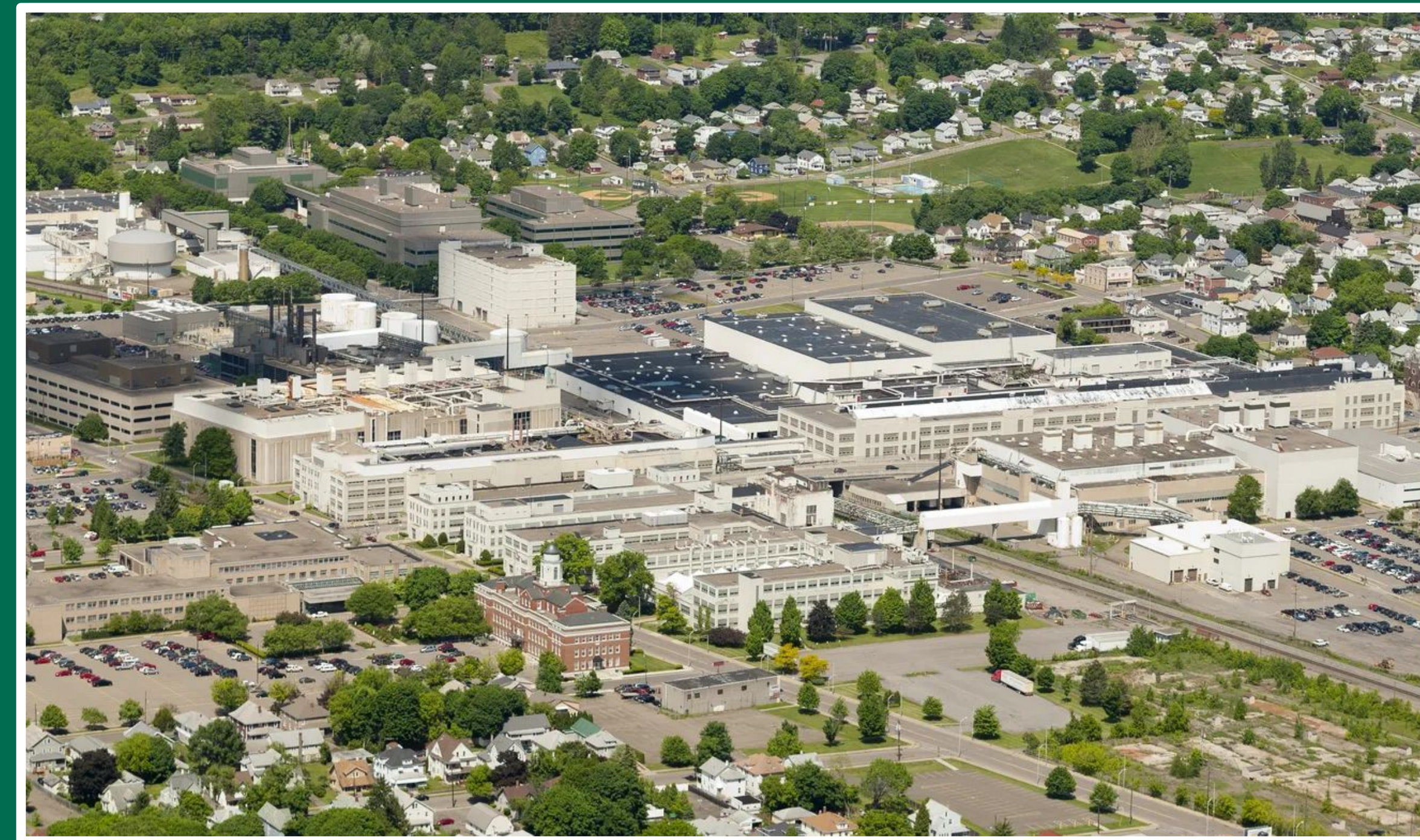
Figure 1 Site to be demolished and redeveloped circa 2014
