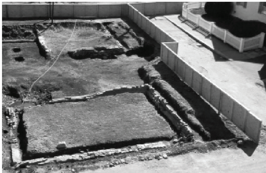
Figure 10. The Paul and Manning wharves excavation (Photo by Martha Pinello, 1993.)
